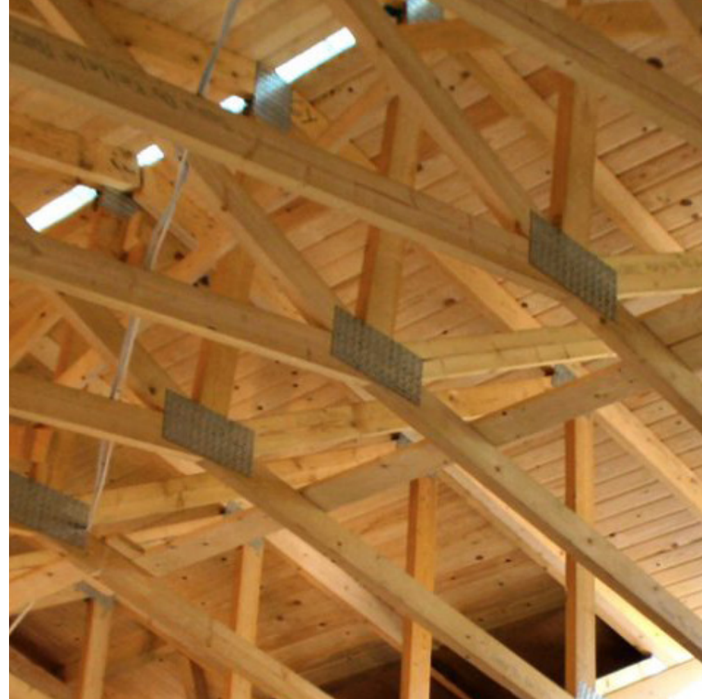
Cut Timber Roofing
