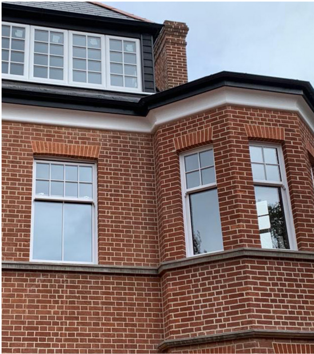
Period Bay Window Replacement
