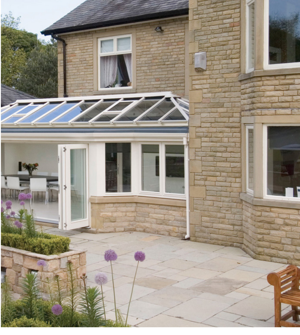
Traditional Conservatory Installation
