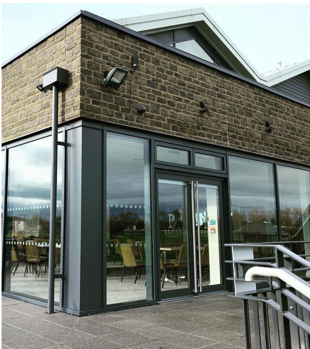
Commercial Glazing Project
