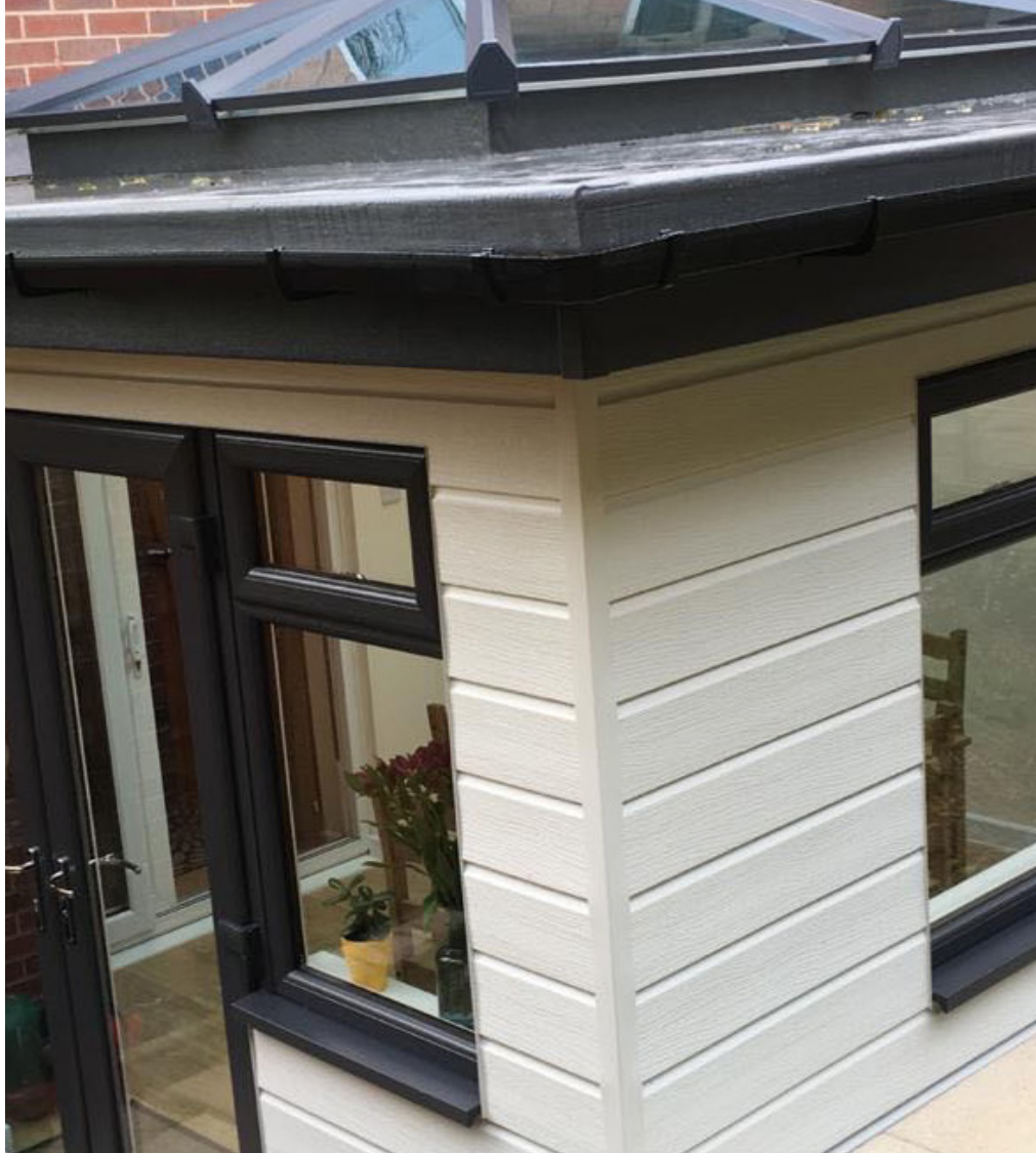
Roofline and Fascia Upgrade
